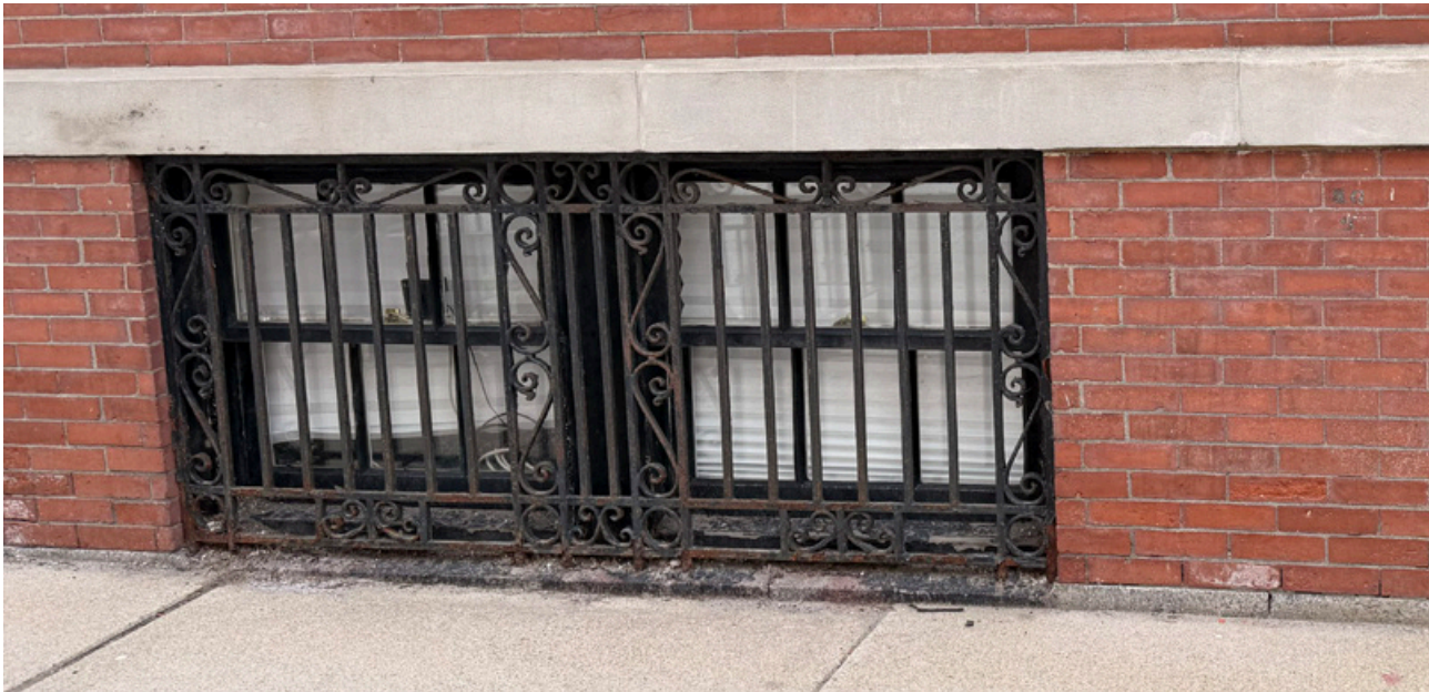
ABUTTER'S GROUND WINDOWS (3 OVER 3)
