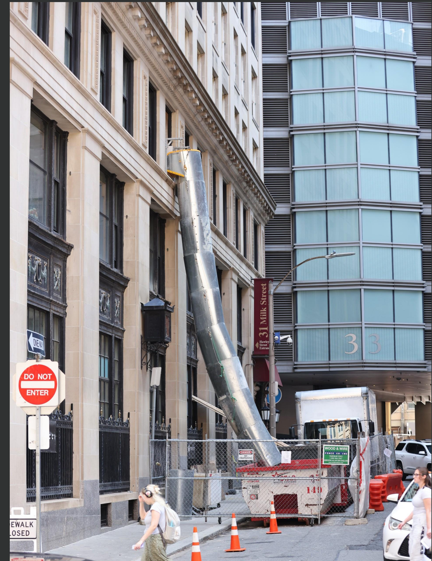
Construction continues at the 31 Milk Street conversion project. The DBA area's nine residential conversion projects have combined to remove nearly 700,000 square feet of office space, substantially impacting the district's office market.
