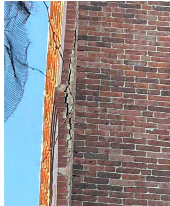
Photo showing masonry bowing and separating from floor framing
