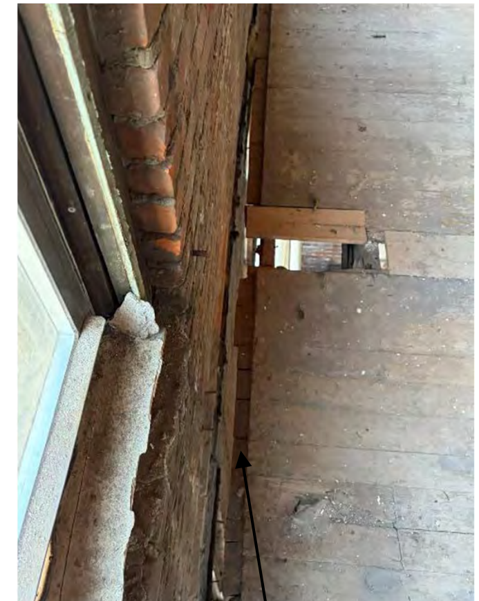
Photo showing masonry bowing and separating from floor framing
