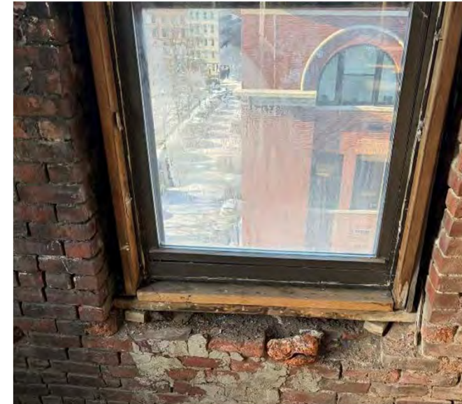
Typical examples of masonry failures
