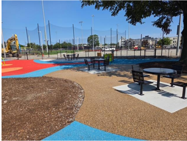
Porous paving/ site furnishings at playground
