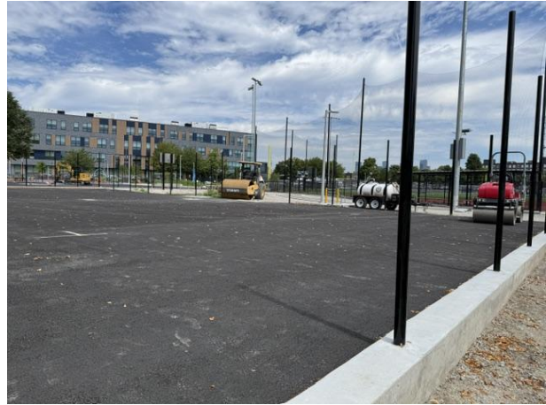
Asphalt paving and fence poles at basketball courts
