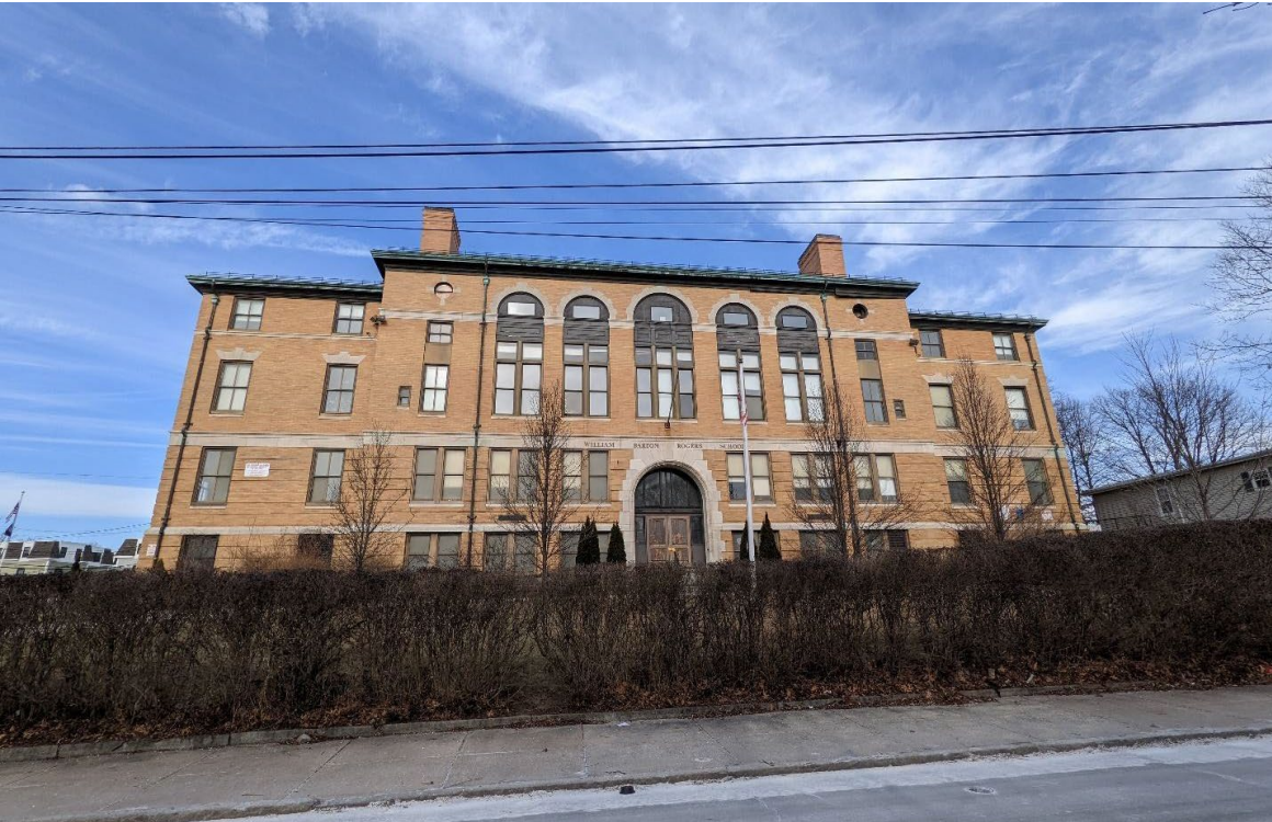
On July 2024, the Hyde Park’s vacant William Barton Rogers School conversion into a vibrant, mixed-income, LGBTQ-friendly senior 75-unit housing development through CPA funding was completed. Source: JM Goldson
