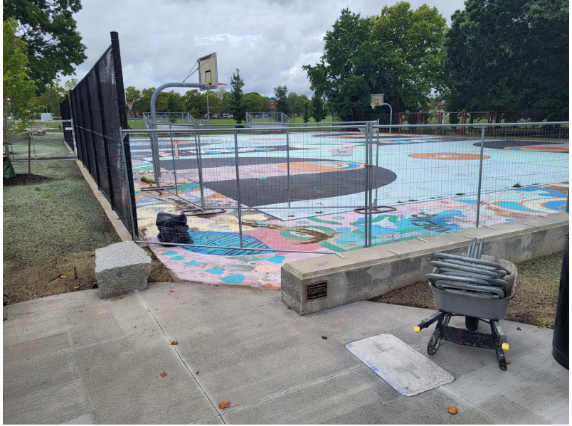
Yellow base plates for the new collapsible bollards (left) and new seat walls (right)
