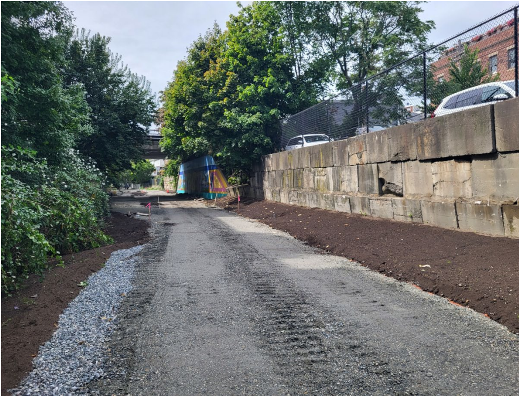
The base material for the future asphalt path
