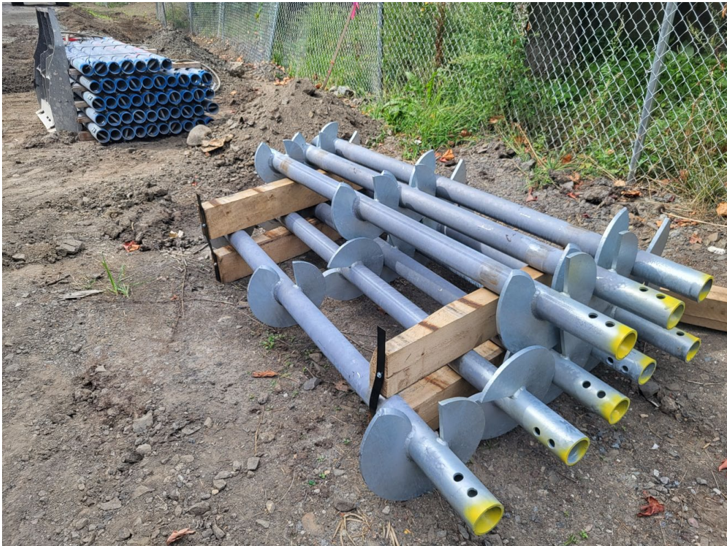
The lead section of the helical pile with blades
