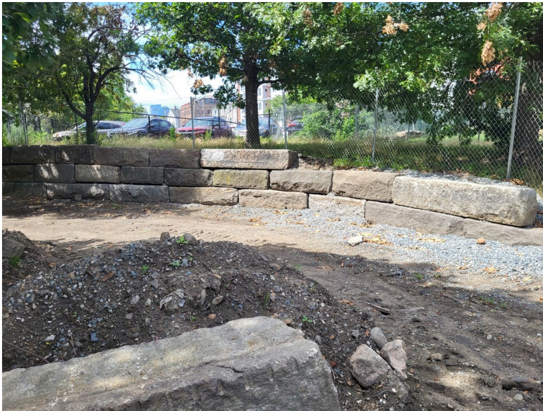
At the Gove Street plaza, the block wall was reinstalled to a greater depth
