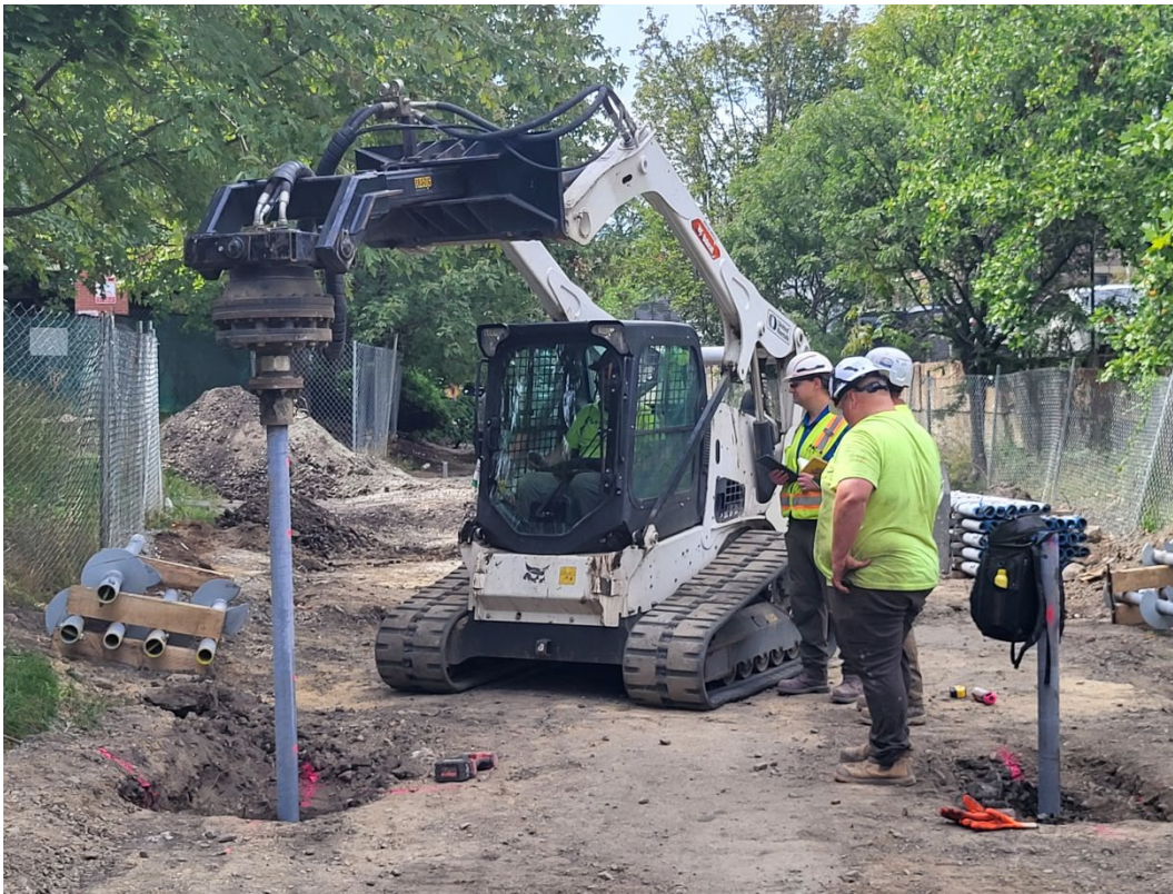
Helical pile being driven in to the ground. The geotechnical engineer records the torque measurement at 1' intervals, which gives them information about the types of soils and loading.
