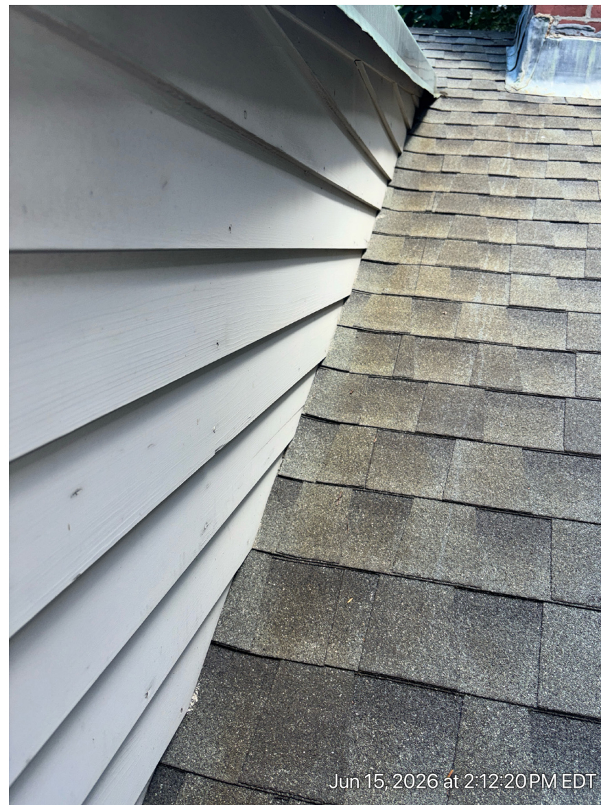
Existing Roofing Material To Be Re- placed In-Kind
