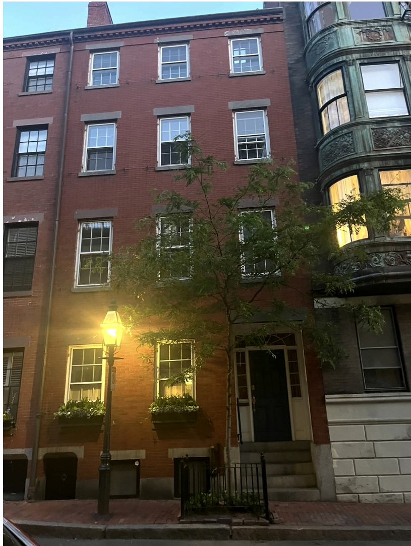
CURRENT STREETSCAPE / EXISTING CONDITION
