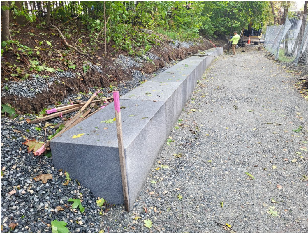
Granite block wall installed along the pathway
