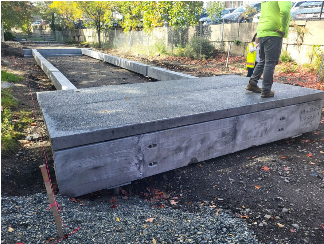
An end section of boardwalk with the decking installed. When the path is installed, it will meet the top of the boardwalk decking flush.
