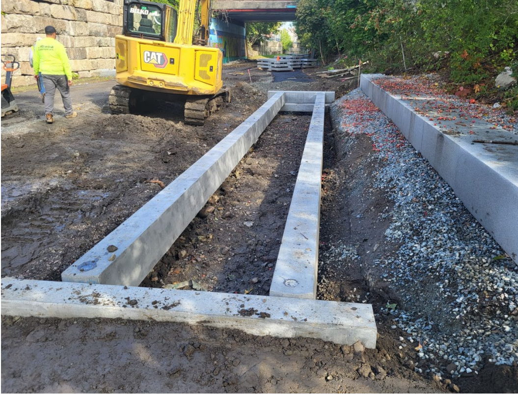
Support beams for one of the boardwalks. Rodent control measures (steel mesh and crushed stone) will be installed under the boardwalks to prevent burrowing.
