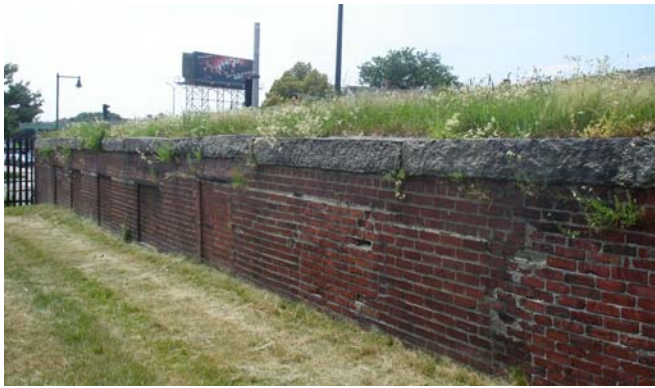
West tombs before restoration
