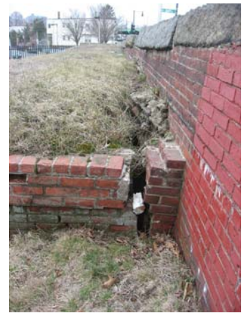
West tombs before restoration
