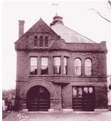
Old Roslindale Fire Station built in 1888 on site of present day Roslindale Branch of Boston Public Library
