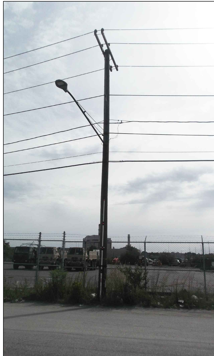
EXISTING PHOTOGRAPHIC VIEW
