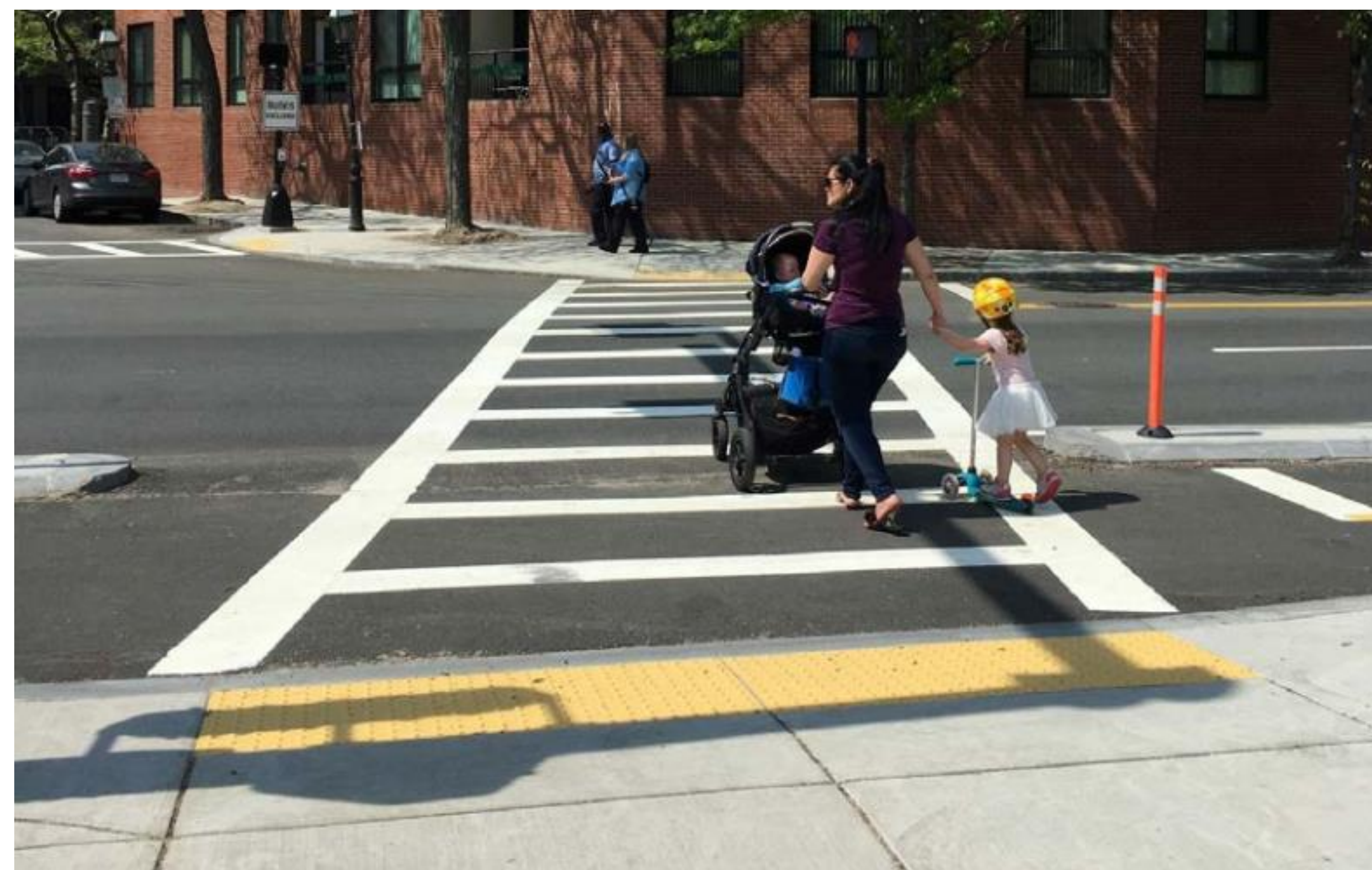
Curb Ramp (Boston)
