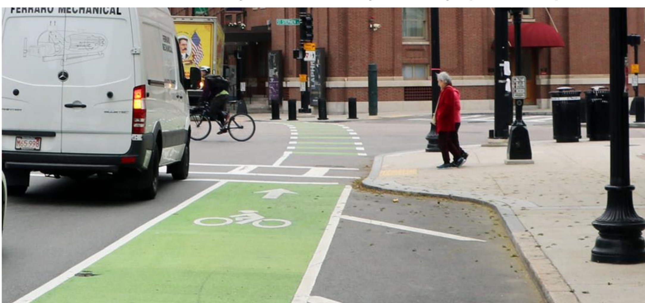
Curb Extension and Bike Lane (Massachusetts Ave.)
