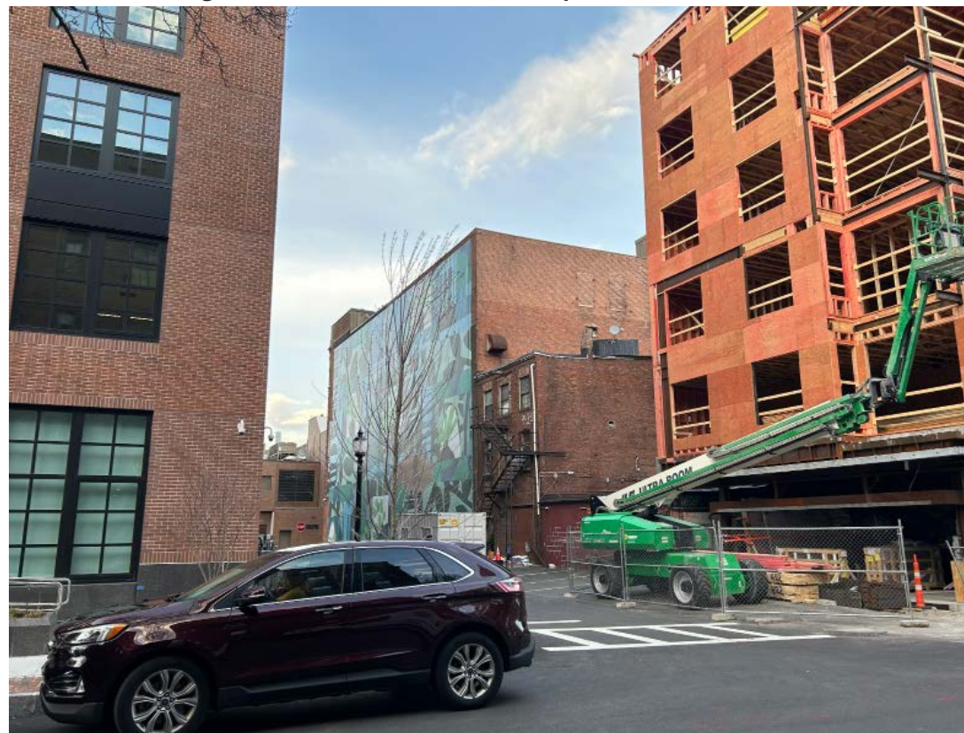
View Looking East on E Canton
